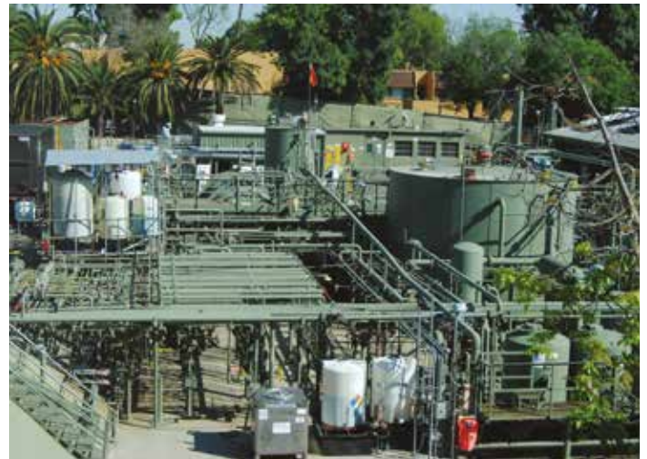
Murphy Drill Site with multi-family apartments in the background.
