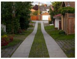
Example of green alley with driving strips that provide functionality, while still allowing for vegetation to be integrated into alley design. Photo Credit: Ben Nelms, National Post
